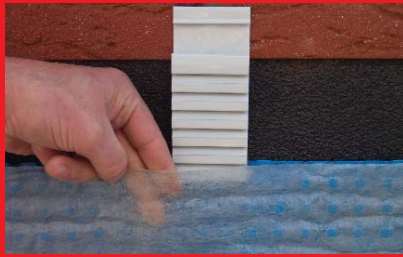
Slip the DS Protection Sheet under the clip.
