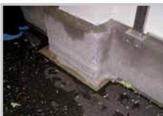
*Far from waterproof: porous floor to wall joint and poor coving.*
