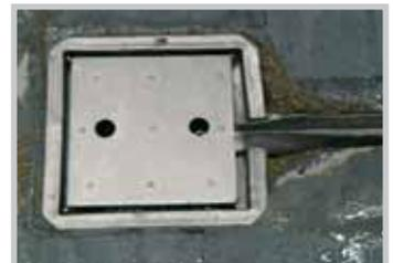
*Consequences of infiltration with spalling around the drains, which can put hygiene at risk.*
