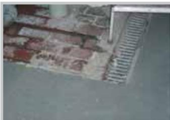
*These conditions can allow infiltration underneath damaged old coatings.*
