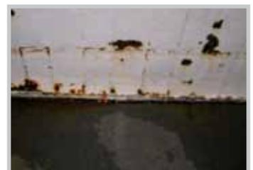
*Water infiltration leads to corrosion and damage.*
