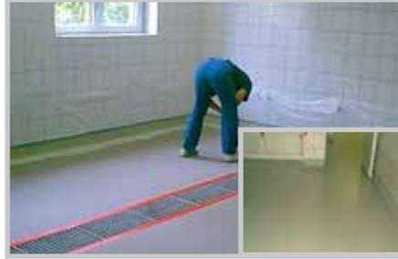
**Only four hours later: Finishing with the resistant top sealing coat**
