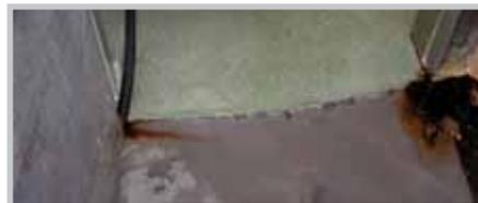
Defective expansion joints and broken edges soon become trip hazards.
