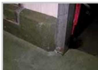
*Impact damage (e.g. due to heavy fork lift traffic) puts hygiene at risk.*
