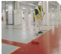
**Requirement:** A non-slip (R 12 standard) coating which can easily be applied with a roller. There will be no labour intensive broadcasting of quartz sand followed by removal of the excess.
