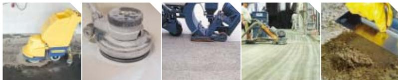
Cleaning, e.g. to remove dirt from non absorbent substrates    Blastcleaning, e.g. on soft substrates or to level rough substrates    Blastcleaning, e.g. to open the pore structure of dense substrate    Grinding / planing, e.g. to remove old non load bearing surface finish layers    Repair blemishes and spalling
